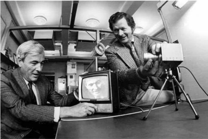
Bell Labs researchers Willard Boyle (left) and George Smith (right) with the charge-coupled device, which transforms patterns of light into useful digital information and is the basis for many forms of imaging, including camcorders and satellite surveillance. Photo taken in 1974.
